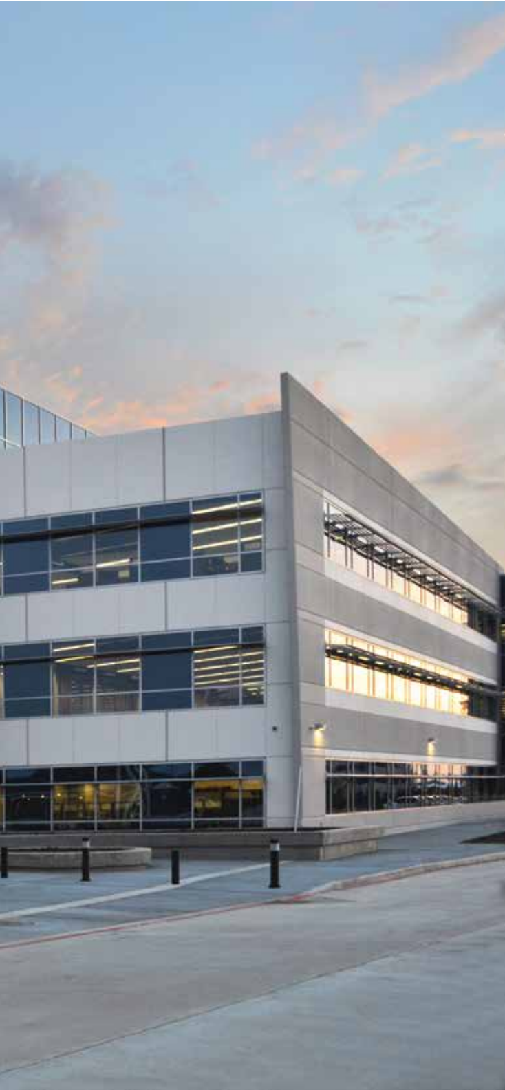
View of entrance to new Administrative building.
