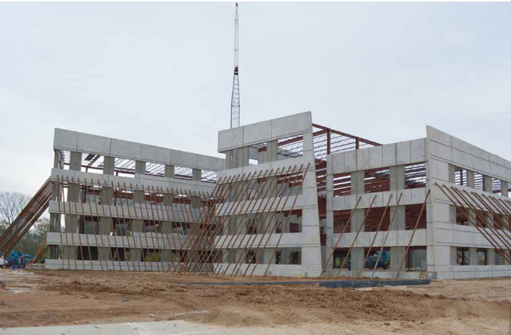
Construction photo of braced Tilt-Up panels following panel erection.
