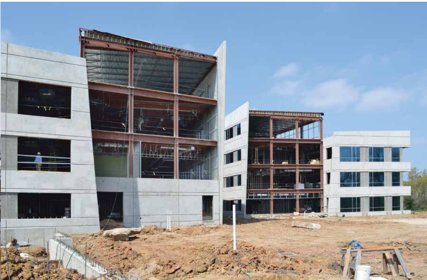
View of hybrid steel and concrete panel structure during construction.
