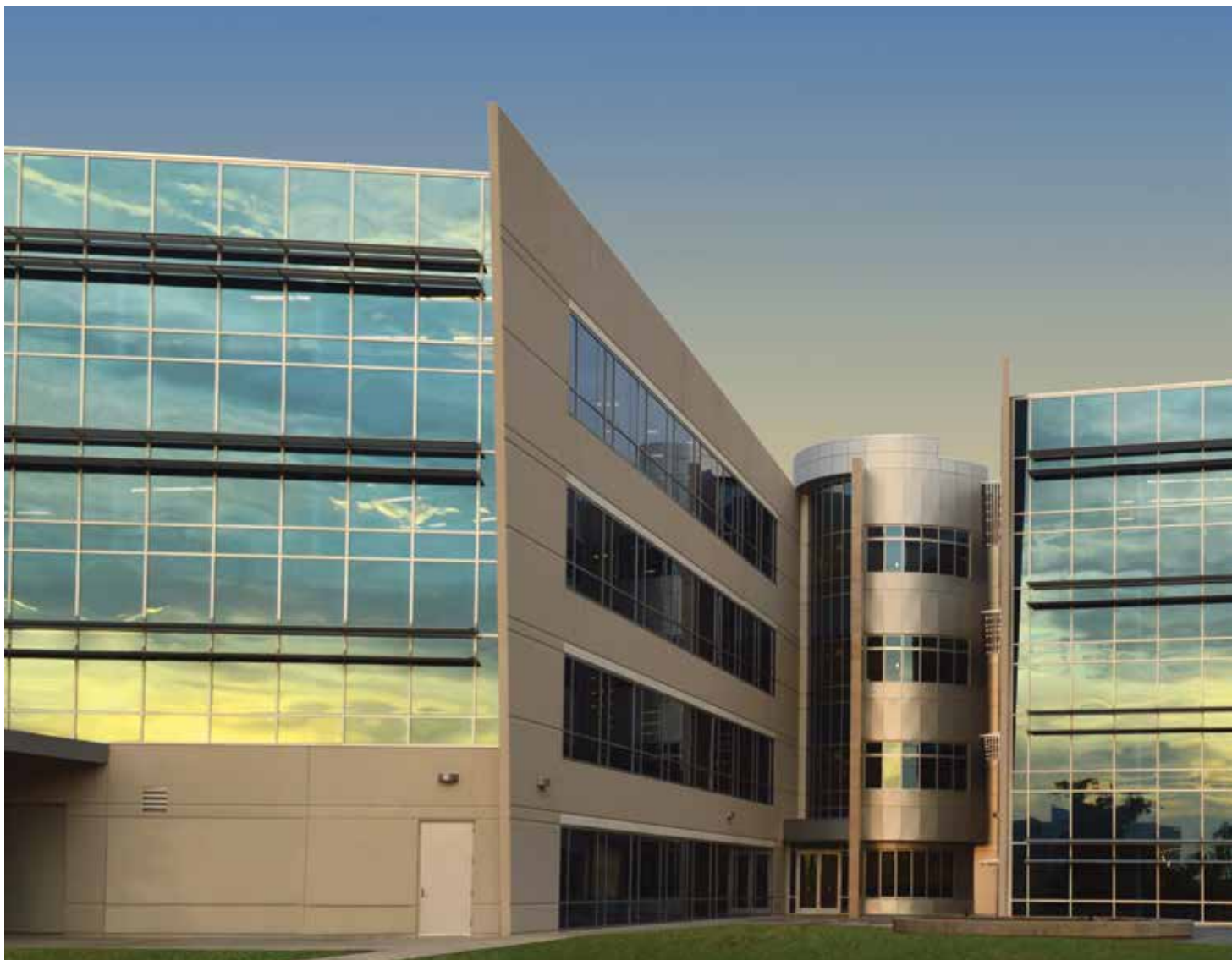
View of four-story panels at East building elevation.
